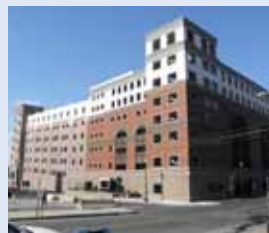
Chestnut Street Parking Facility West Chester, PA Submitted by The Harman Group
