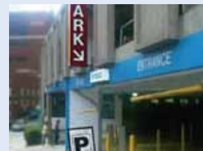
Chatham Center Parking Garage Pittsburg, PA Submitted by PSx
