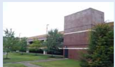
Chubb and Son Parking Garage Whitehouse Station, NJ Submitted by Wardle Engineering
