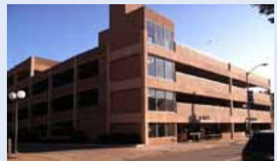
East 8th Street Garage Erie, PA Submitted by Roth Marz/Erie Parking Authority
