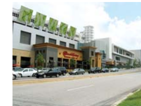
Addition/Improvement: Towson Town Center Garage Expansion Towson, MD Submitted by Timothy Haahs & Associates, Inc.
